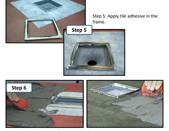
Step 6: Apply two layers of Tanking membrane
